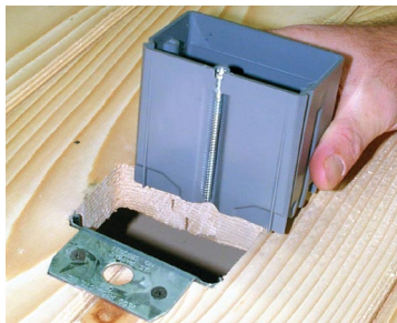
Install clip over subfloor.
